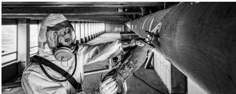
Asbestsanering in 2015 (Chris Pennarts)
